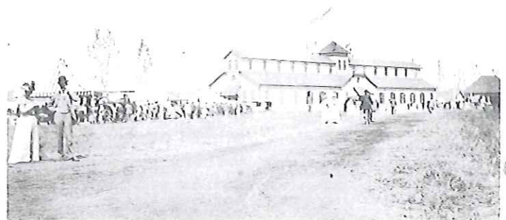
The committee acquired 28 acres from A. G. Tuite for the fair grounds. Maps show the grounds were on the north side of Railroad Ave., between Bridge St., and North St.
